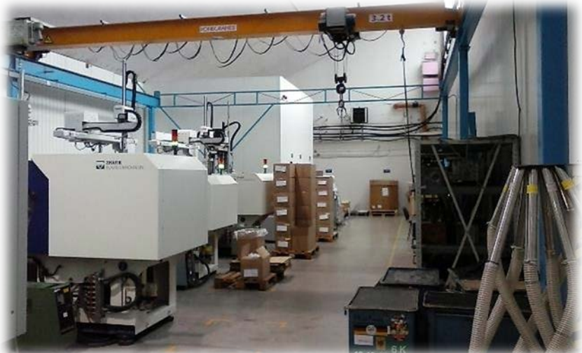
small shop, cooling system
